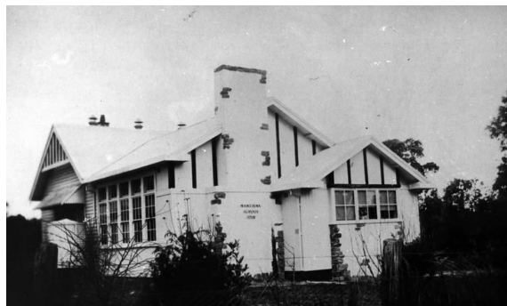
Above: More recognisable Wantirna State School brick building showing the number 3709 on the chimney. (Knox Historical Society image)
