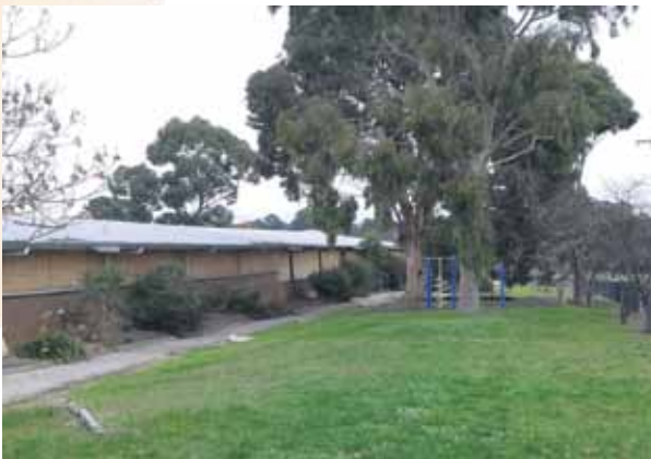
Wantirna Heights Primary School under demolition
