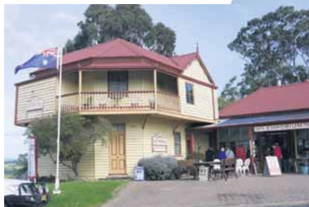
Bates Emporium General store, Wallaga Lake, NSW
