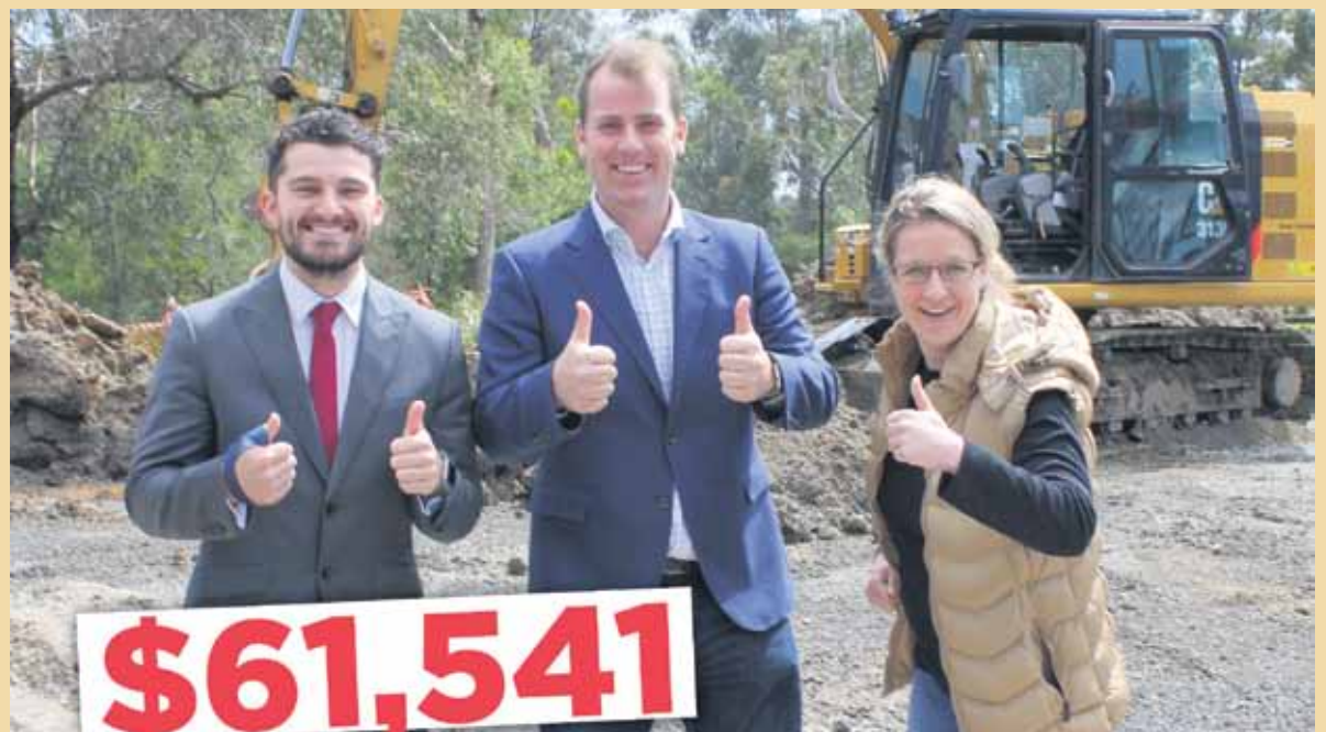
Cr. Jake Keogh (as Knox Mayor), Jackson Taylor MP and Cr. Marcia Timmers-Leitch celebrate the announcement of brand new solar lighting at Marie Wallace Reserve in Bayswater.
