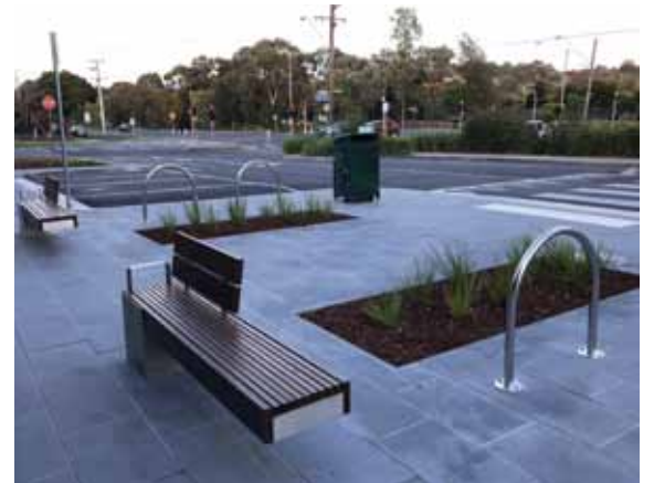
Completed Studfield Shopping Centre Car Park
