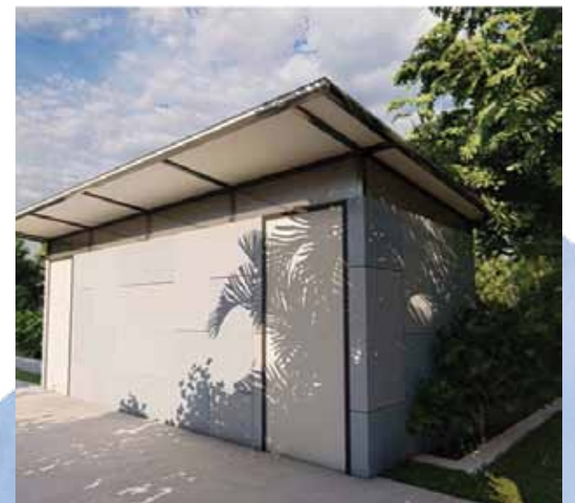
New toilet block - photo provided by Cr. Lisa Cooper
