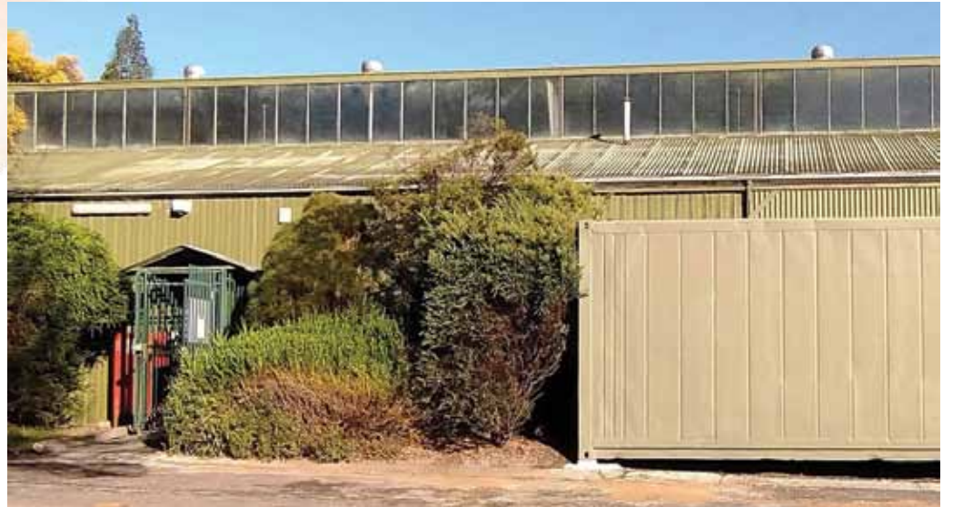
The Museum's entrance showing part of the new shipping container.
