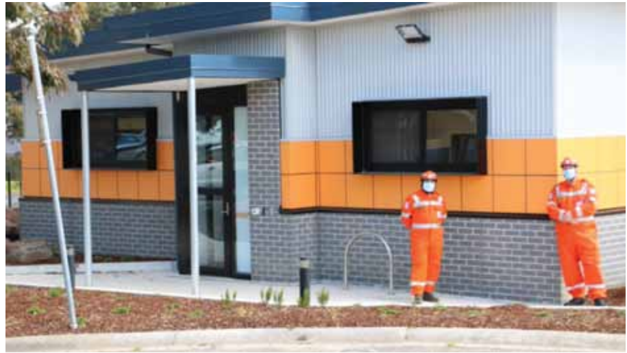
The New VICSES Knox facility in Knoxfield - photo sourced via https://www.facebook.com/SESKnoxUnit
