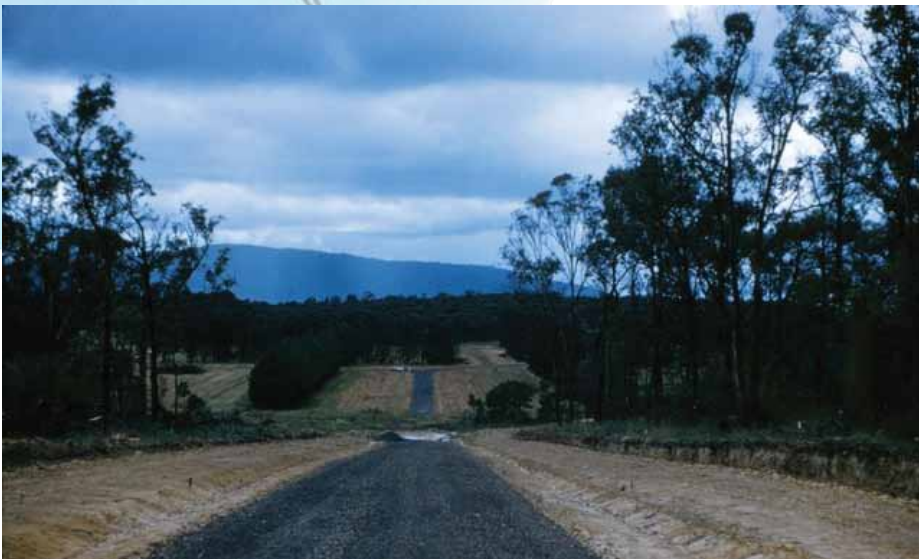
December 1959 - Looking down the hill at Eastern Peak estate, Wantirna Vic
