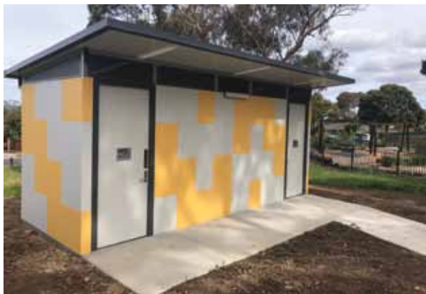
Templeton Reserve Public Toilet
