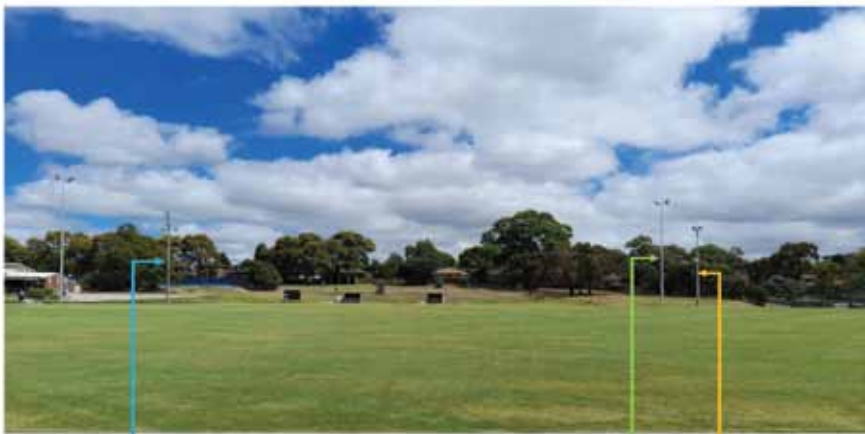
At Templeton Reserve there are a number of other light towers and one other telecommunications pole shows here. There is no change proposed to these poles.
