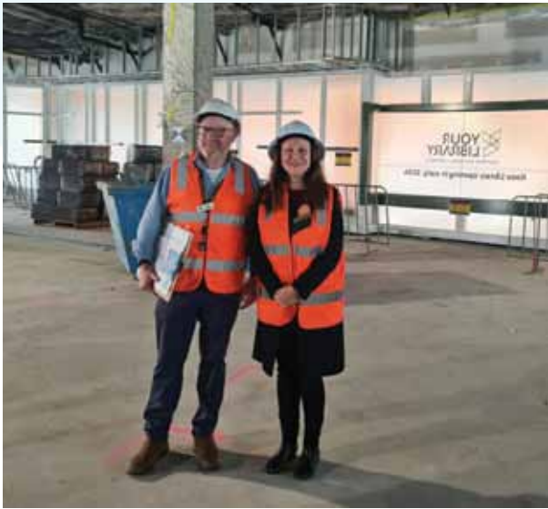
Knox Library Construction
